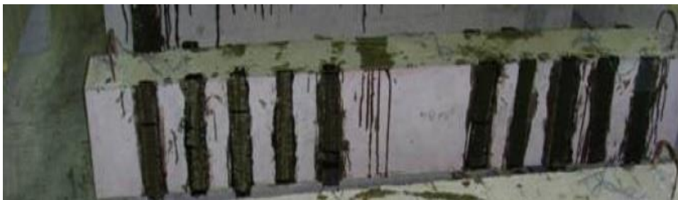
Figure 6: Beams strengthened with vertical strips (Group-2). (Nadeem A. Siddiqui 2009)
