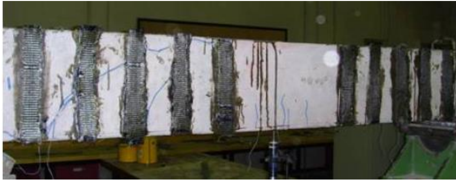
Figure 23: Crack pattern for strengthening RC beam, group-2_ (Nadeem A.S 2009). (Experiments)
