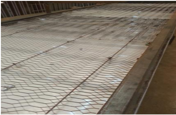
Figure 4: Expanded Metal & 4R6 Bars Reinforcement Placement
