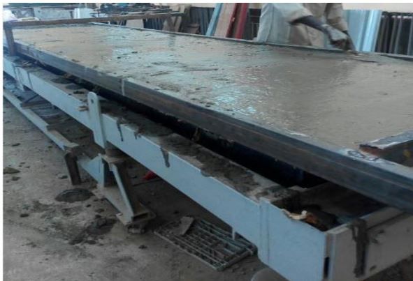
Figure 5: Compaction by Vibration Table
