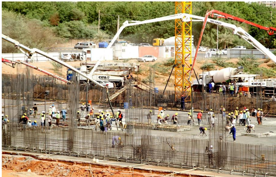
Figure 5: a photograph during the concrete pour
