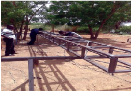
Plate (1): Assembly of Lattice Box Girders.
