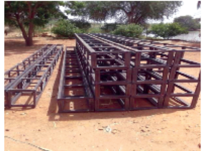
Plate (2): Lattice Box Girders ready for lifting.
