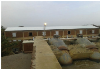
Plate No. (10): Side View of CMS roof upon completion.
