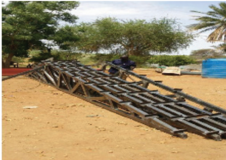
Plate No. (6): Steel Truss ready for painting & lifting.
