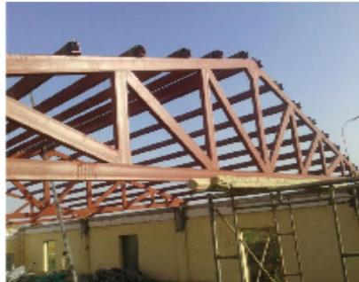
Plate No. (7): Steel Truss fixed to position together with purlins.
