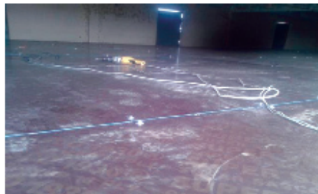
Plate (5): View of overhead platform from above
