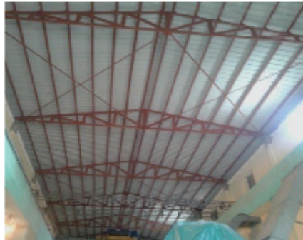
Plate No. (9): Complete CMS roof after removal of the overhead platform.
