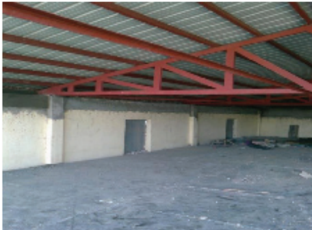
Plate No. (8): Roof Sheeting's fixed on trusses.
