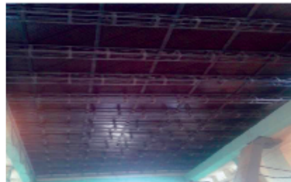
Plate (4): View of overhead platform from beneath.
