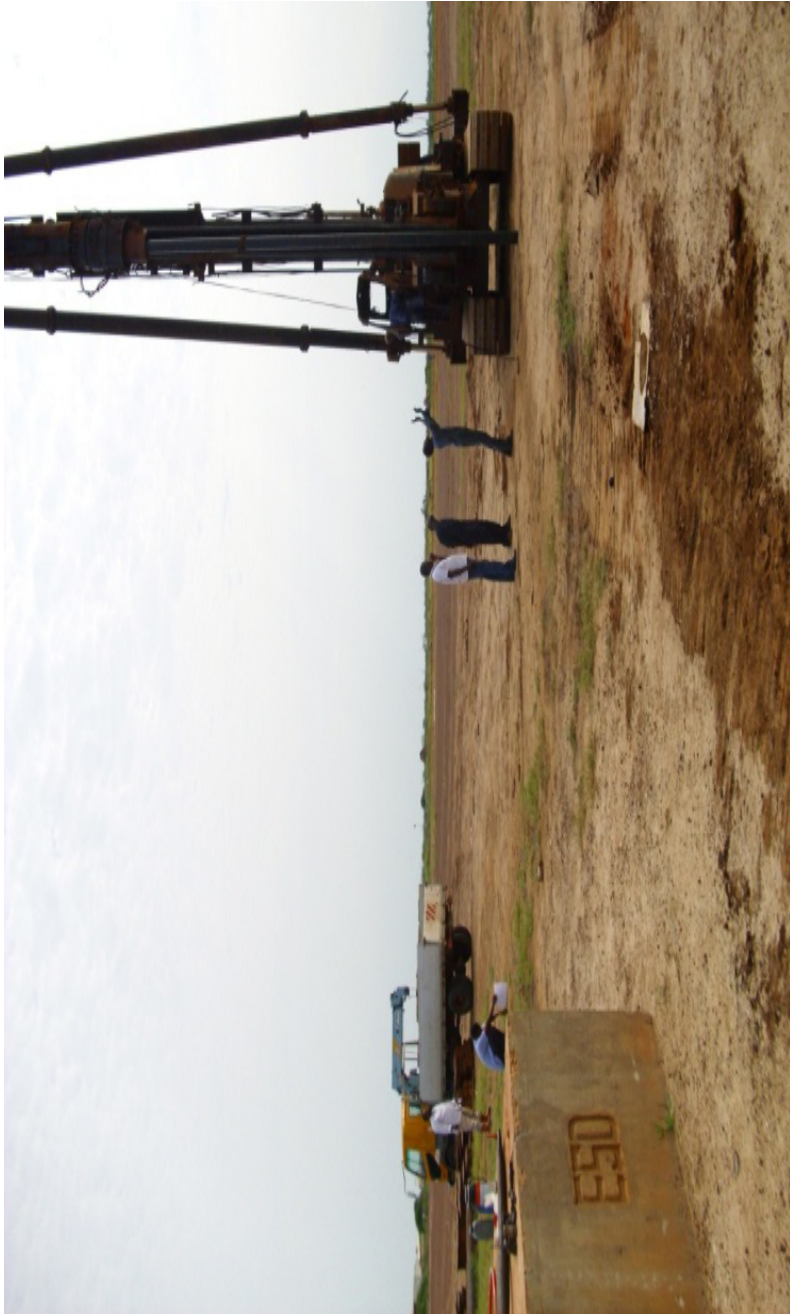
Plate 1: View of the site and the driving system of the steel pipe piles
