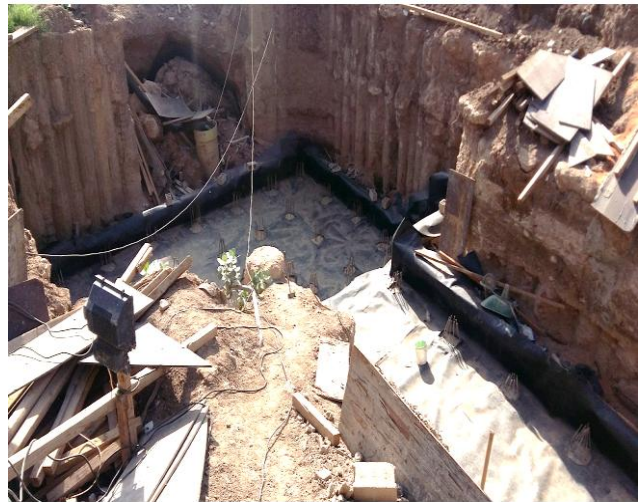
Fig. 8. Falling down of excavation sides after dewatering
