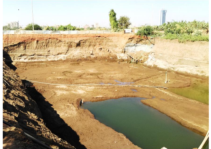
Fig. 10. The project site filled with water before dewatering
