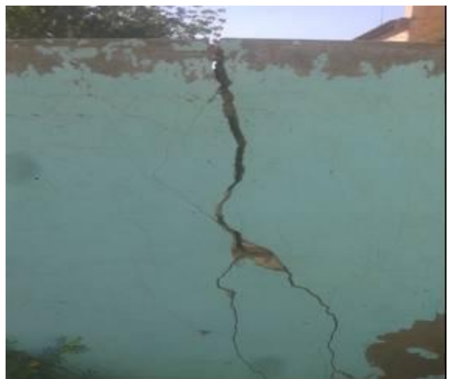
Fig. 9. Serious cracks in walls of adjacent buildings
