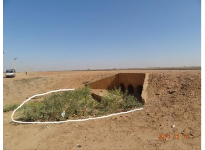
Fig. 3 Scour Hole in Plan View
