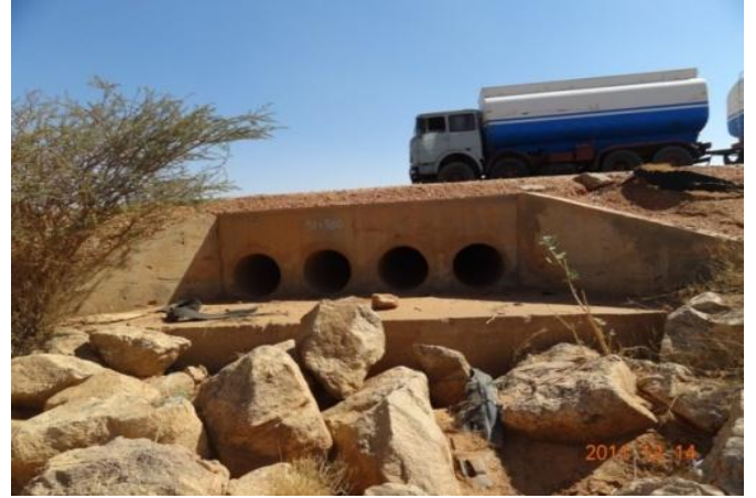
Fig. 5. Post Protection by Boulders after Occurance of Local Scour
