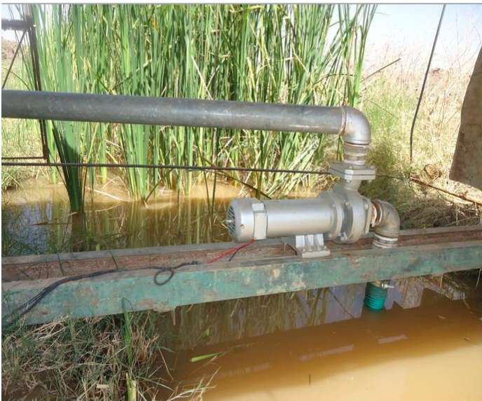
Fig. 10. DC solar electric centrifugal pump
