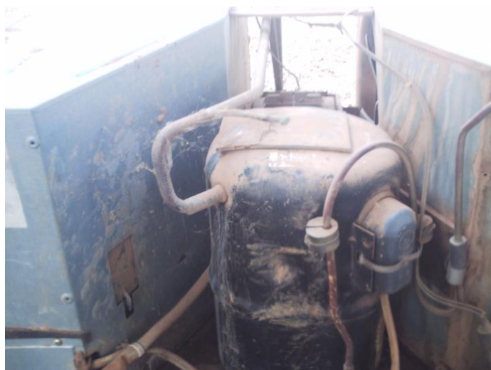
Fig.3. Compressor and condenser coil before cleaning
