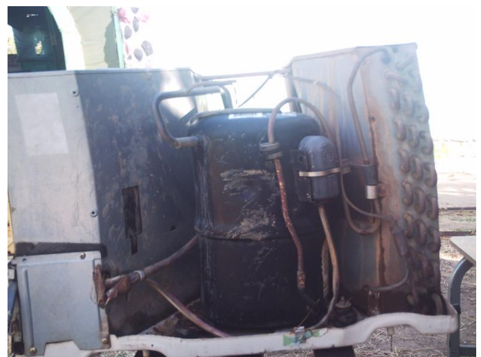
Fig.4. Compressor and condenser coil after cleaning
