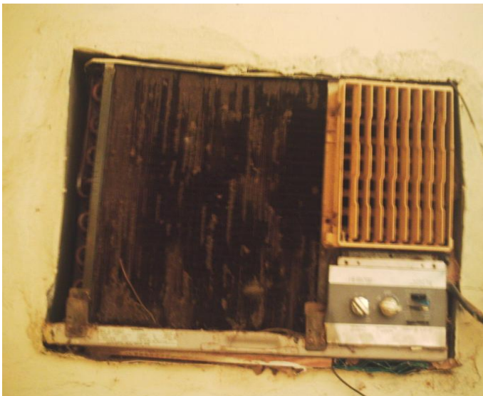
Fig. 1. Evaporator coil before cleaning
