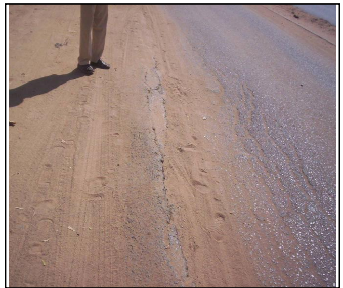
Plate (1): Severe distresses of potholes and rutting appear on Alazhari Road surface
