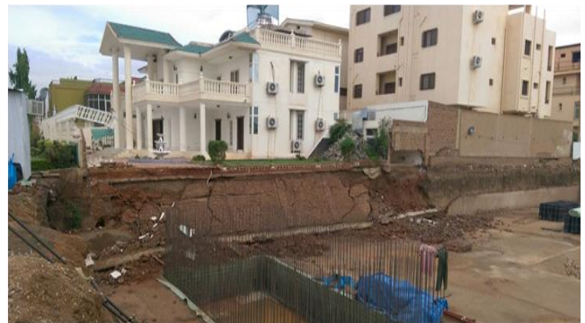
Fig.9 The Shoring Piles Distributed All Around
