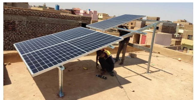
Fig .8. 1.82 kW p off-grid rooftop PV system without power bank during installation in the Abo-Adam district, Khartoum
