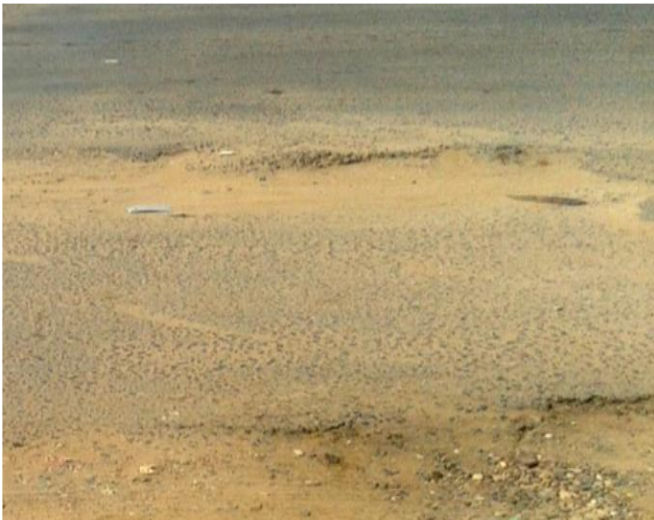
Fig. 5: Dangerous potholes and edge failure of road (R4)
