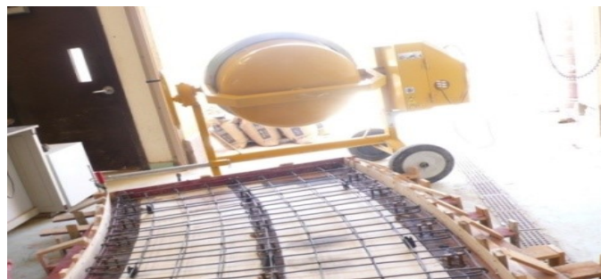
Fig.7. Distributions of Reinforcement and Form Work
