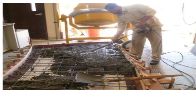
Fig.8. Placing Fresh Concrete
