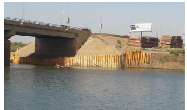
Fig8: Sheet pile installed around the abutment
