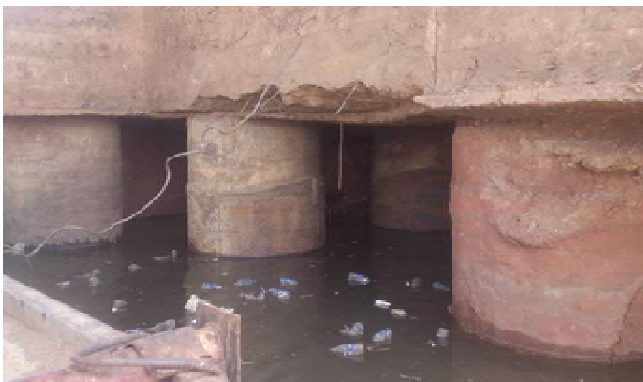
Fig6: The foundation piles surrounded by water
