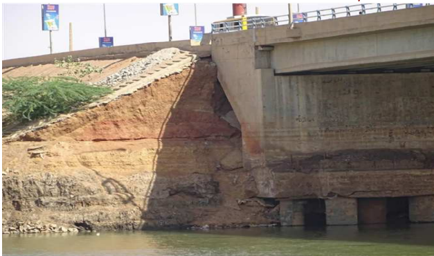
Fig5: Excessive scouring occurred around the east abutment
