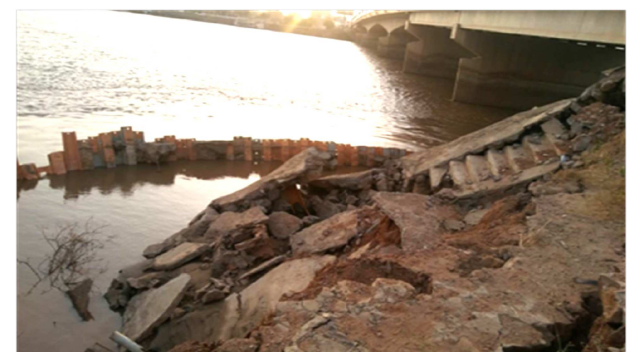
Fig.9. Serious failure and collapse of the protection around the abutment
