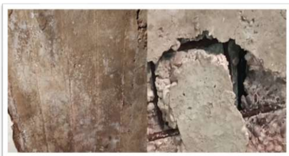
Figure A .9: Spalling occurred in RC slab in room 3
