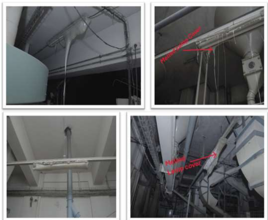
Figure A .7: Melting without ignition of the lamps plastic cover [25]
