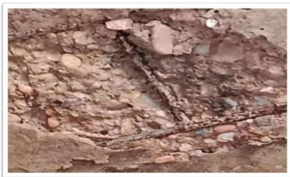
Figure A .9: Spalling occurred in RC slab in room 3
