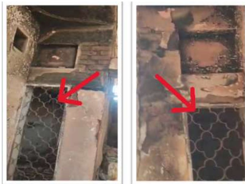
Figure A.12: Metal grill and window frame with soot deposit with no distortion
